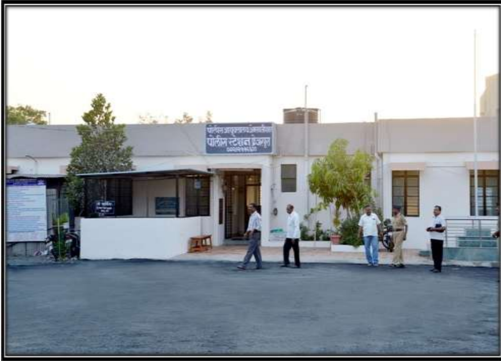
SMART POLICE STATION OF AMRAVATI CITY
